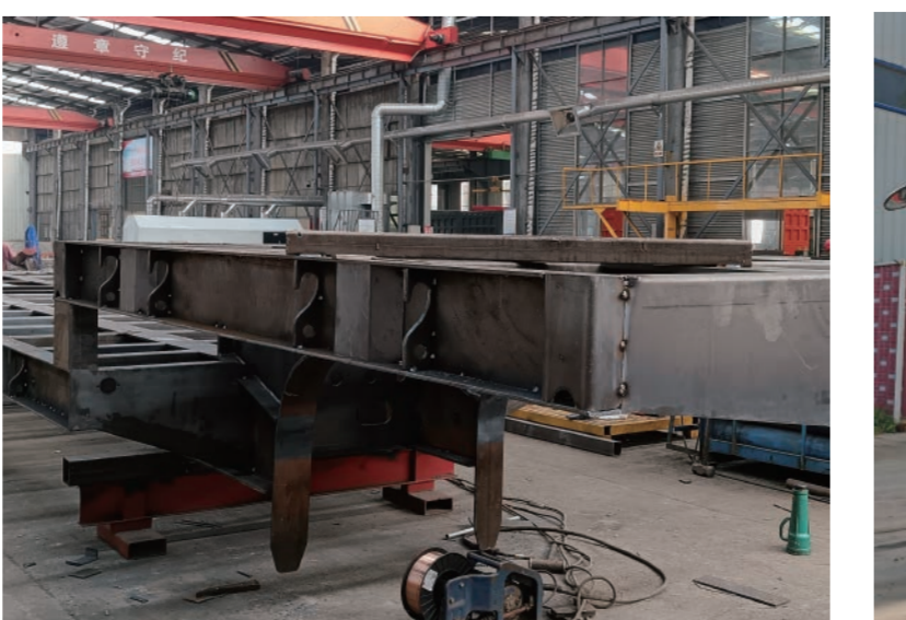
SAND BLASTING AND RUST REMOVAL
